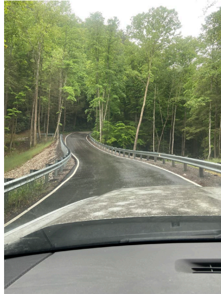
Image 4: KY-715, looking South, road repair a drainage crossing, MP 11.1.
