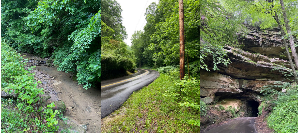
Image 7: Moreland Branch. Image 8: KY-77, looking East. Image 9: Western entrance to Nada Tunnel
