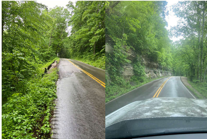
Image 5: KY-715, looking East, slide repair with rails, MP 2.2
